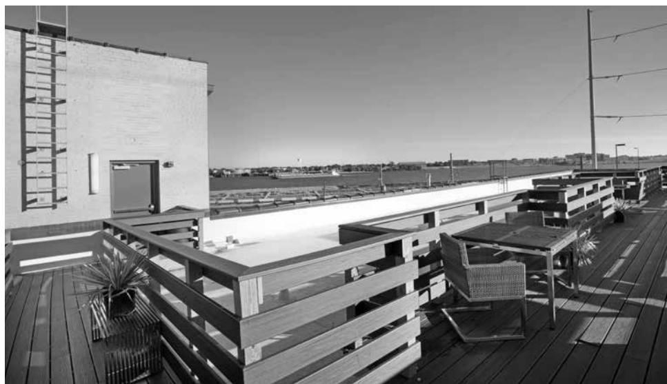
Centennial Place roof
