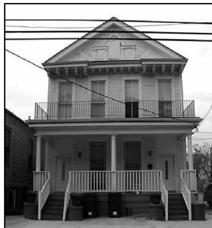
An energy efficient house increase airflow between rooms. It also included work-intensive solutions such as insulating the underside of a roof with spray foam.
